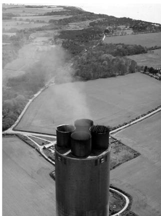
*Blue and white smoke is evidence of SO<sub>3</sub> present in the stack gas as condensed sulfuric acid. Monitoring of opacity (while useful) will not reveal the underlying problem.*
